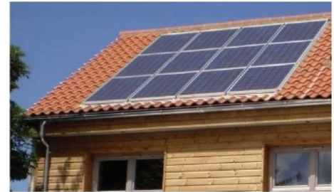
working on pioneering eco builds
