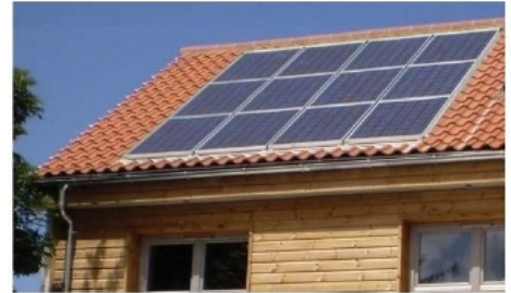
working on pioneering eco builds
